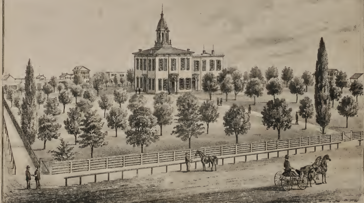
HANCOCK COUNTY COURT HOUSE, CARTHAGE, ILL.
